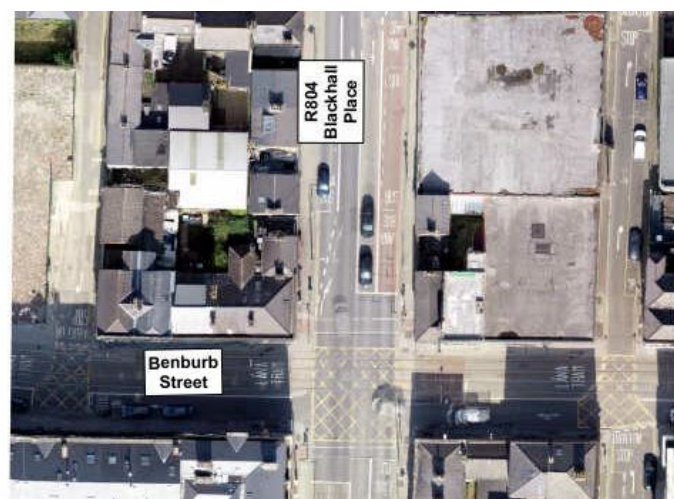
Image 5.41: Blackhall Place / Benburb Street Signalised Junction
