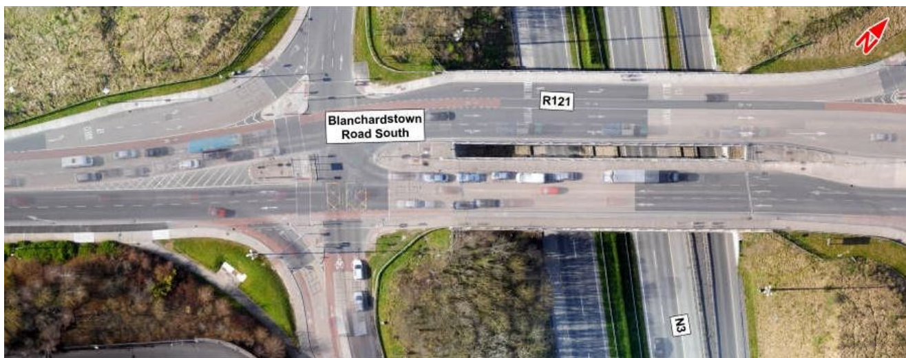
Image 5.5: R121 Blanchardstown Road South / N3 off-slip Signalised Junction
