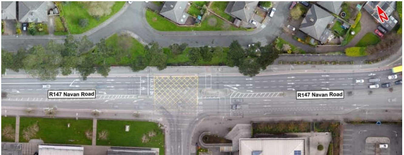
Image 5.28: R147 Navan Road / Cabra Library Signalled Junction
