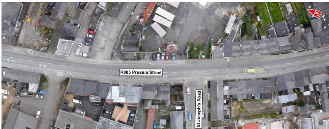
Image 5.35: R805 Prussia Street / St Joseph's Road Priority Junction
