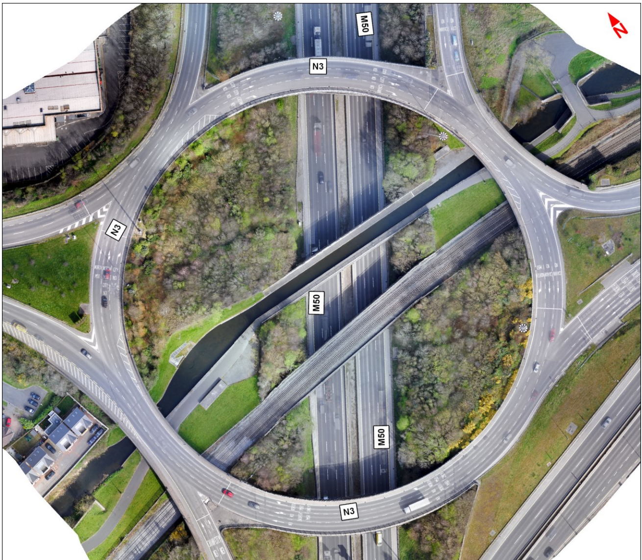
Image 5.16: N3 Navan Road / M50 Junction 6 Interchange
