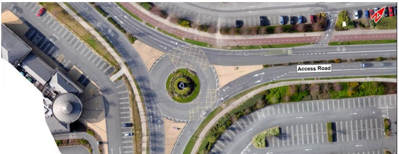
Image 5.9: Access Road / Access Road South Roundabout
